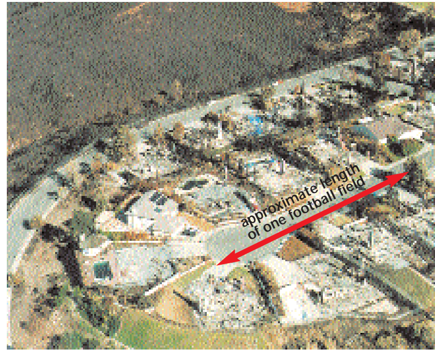
Wildfire attacked this neighborhood with a vengeance. Driven by Santa Ana winds, it raced through homes at rates even faster than the fuel examples at the right—growing by more than 8 football fields per minute.
